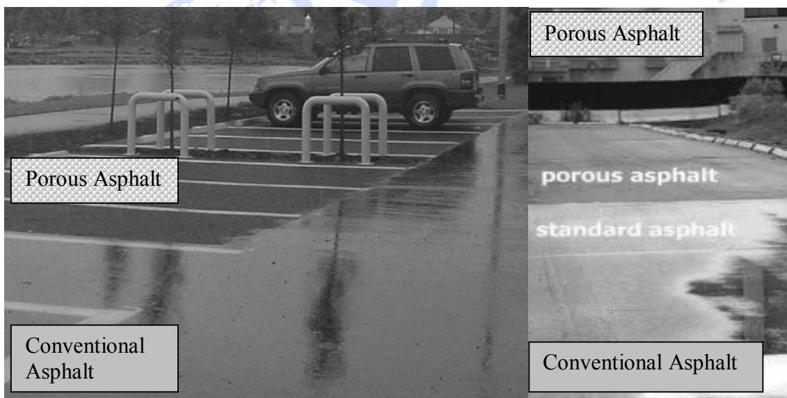
Fig.2. Anti- aquaplaning effect of porous asphalt pavement.
